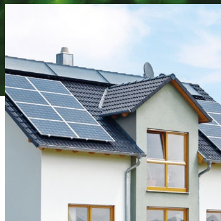
PHOTOVOLTAIC MODULES AND INVERTERS
